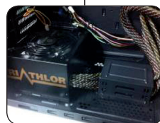
To support bottom cable routing
